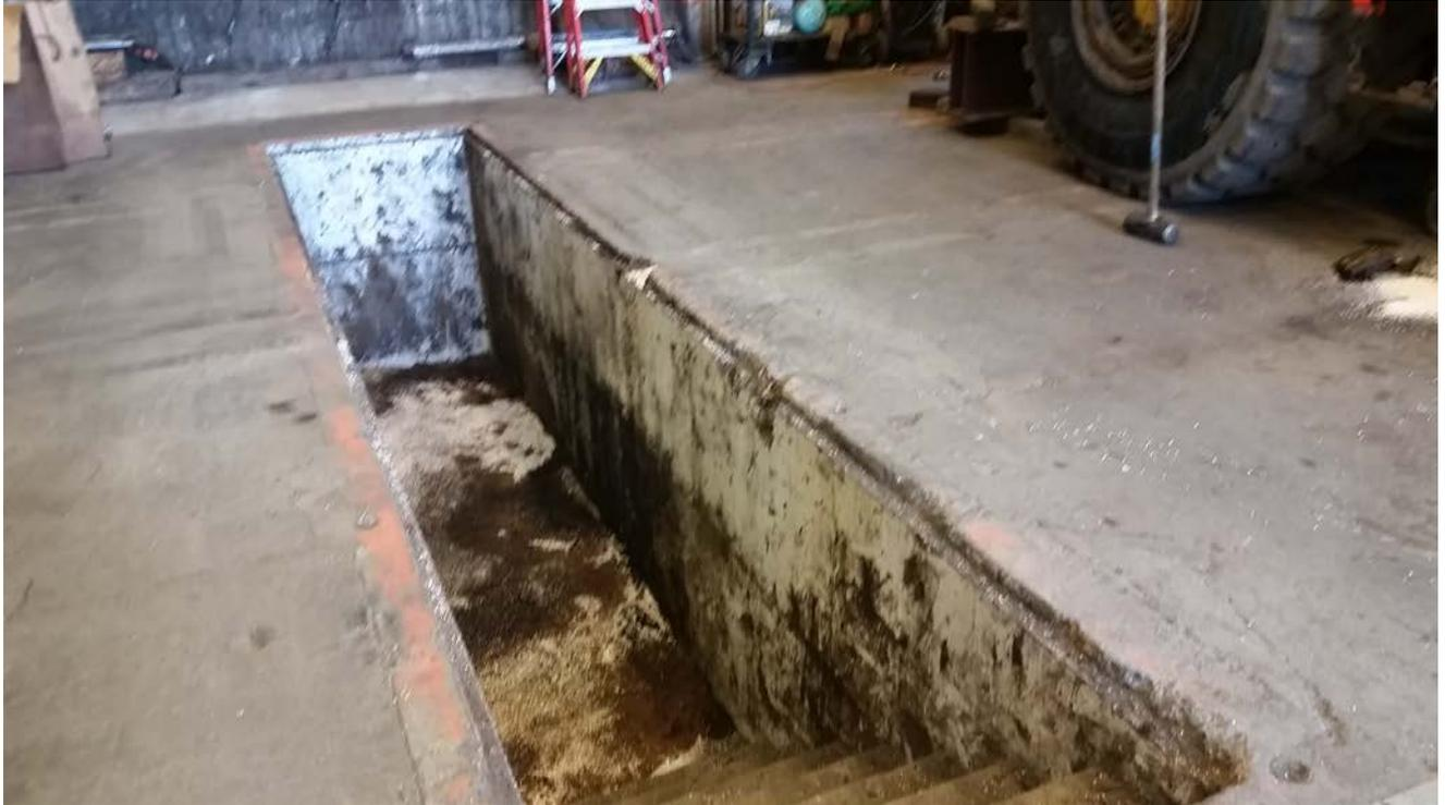
**Photograph 21:** Significant staining in maintenance pit inside West-Central Maintenance Building.
