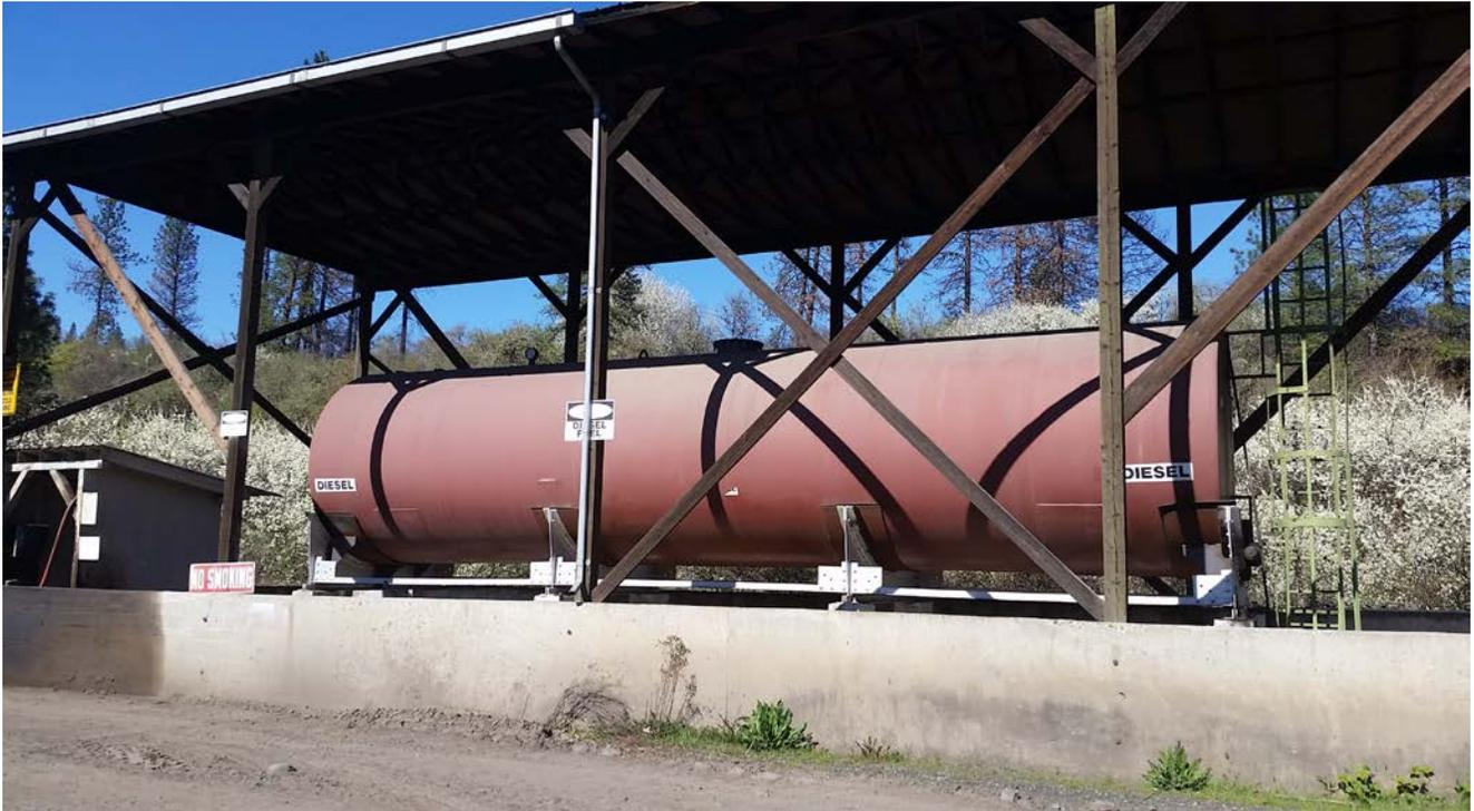
**Photograph 7:** Twelve-thousand-gallon diesel AST, with significant staining.
