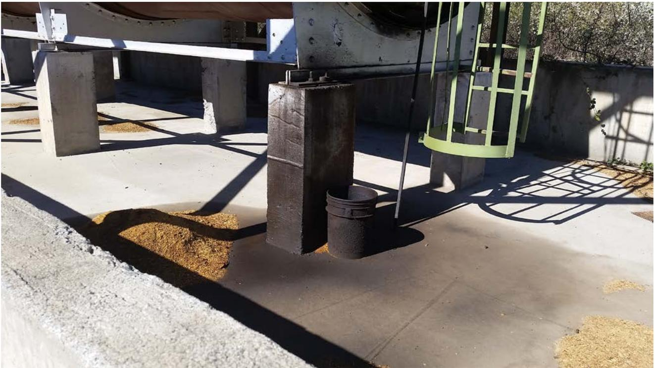
**Photograph 6:** Inside bermed area of 12,000-gallon diesel AST, with significant staining.
