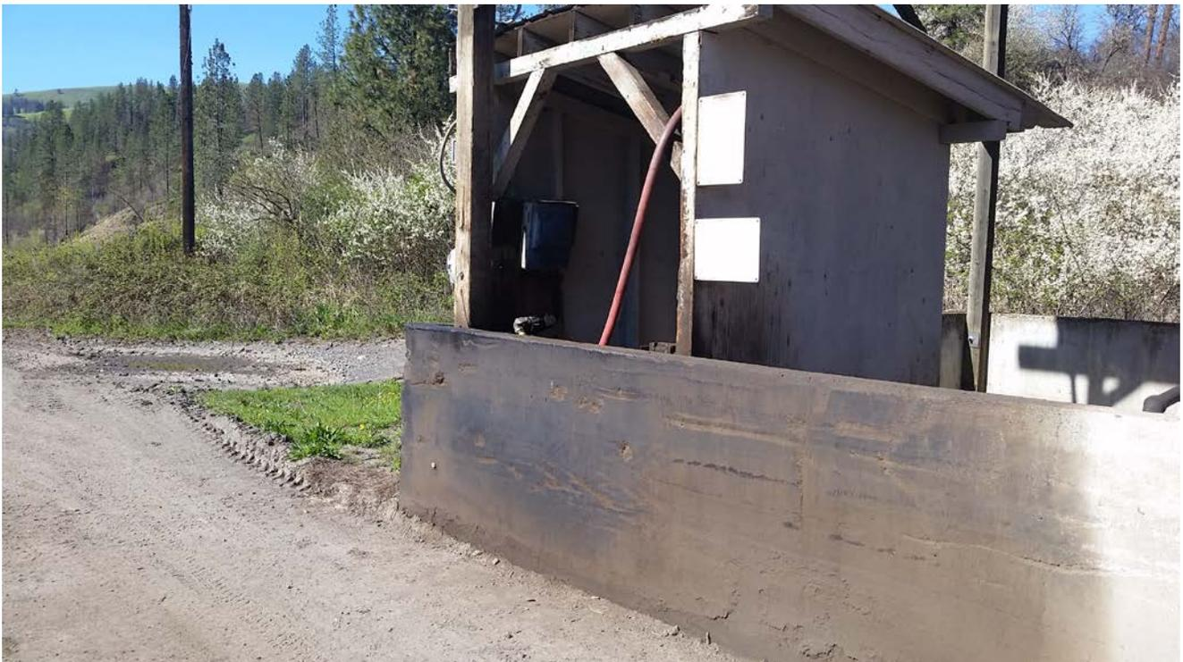
**Photograph 8:** Fuel pump for 12,000-gallon diesel AST, with significant staining.
