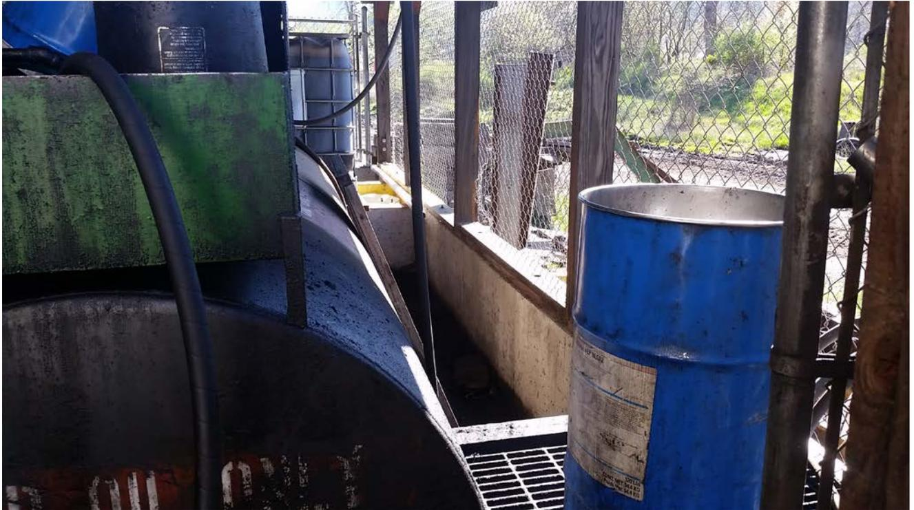
**Photograph 19:** AST, totes, and drum storage adjacent to West-Central Maintenance Building, with significant staining.
