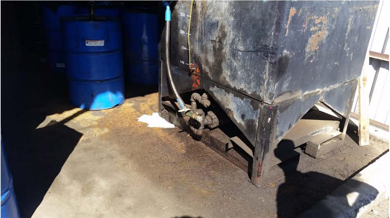
**Photograph 37:** Significant staining inside oil storage building.
