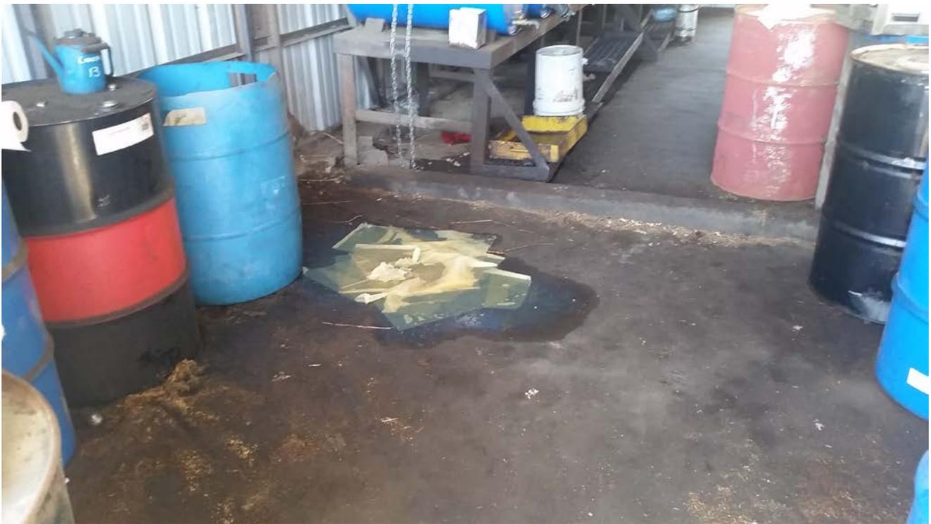
**Photograph 38:** Significant staining inside oil storage building.
