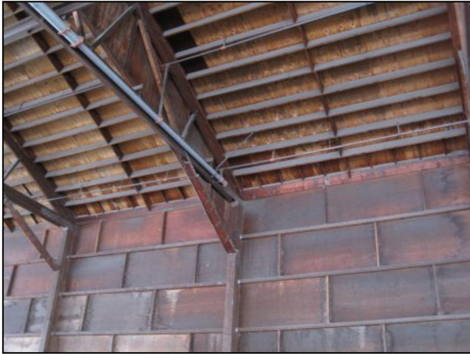
Metal piping on ceiling of Building 4 (fire suppression system).
