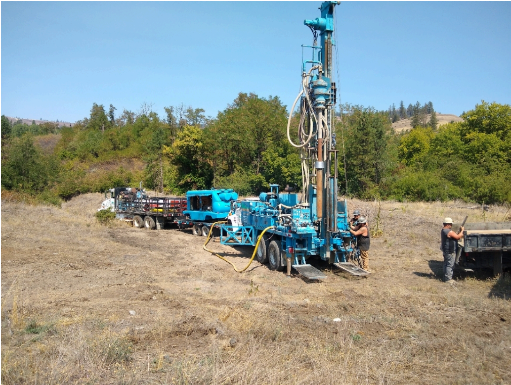
Photo Looking Northeast Photo Description: Drillers setting up at BH-1
